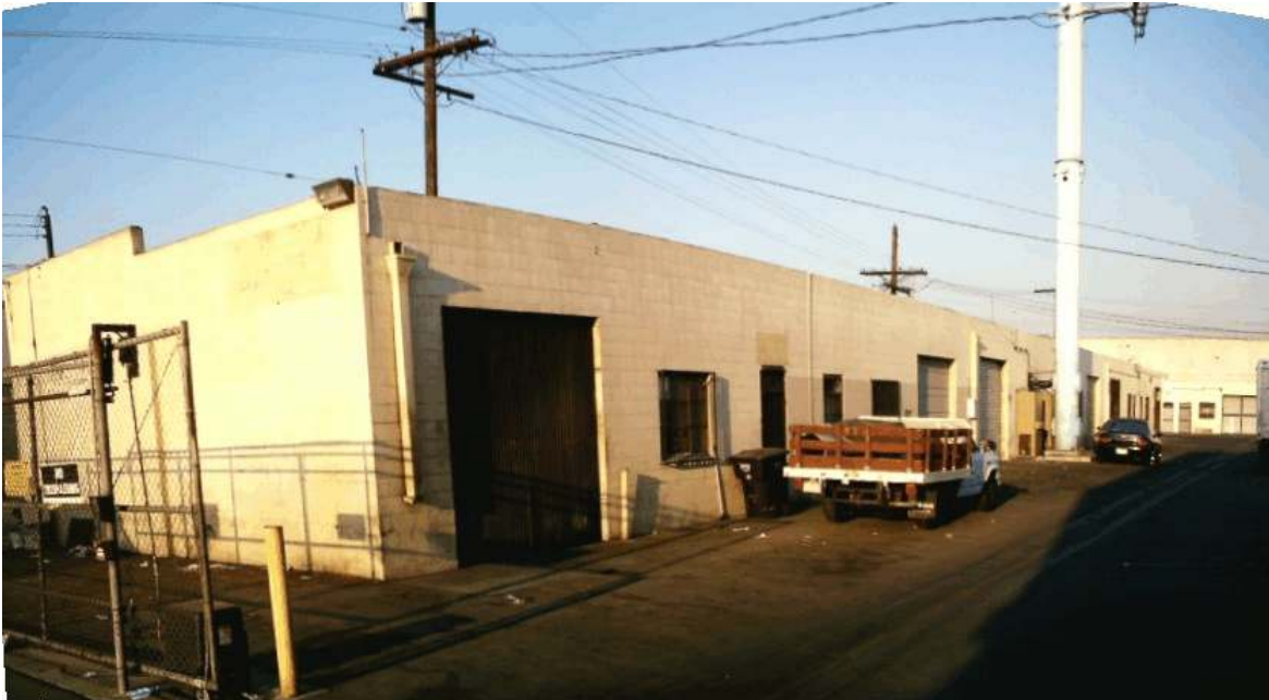
Front View of Structure #4
