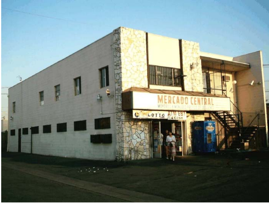
Front View of Structure #1
