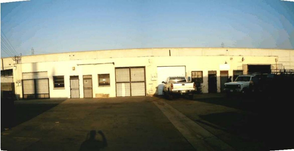
Front View of Structure #3
