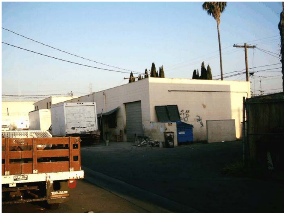
Front View of Structure #2
